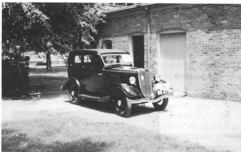
"WG in front of the workshop, now in Greenfield Village, but which was originally located behind 58 Bagley Street in Detroit and in which Henry built his first car, the Quadricycle, in 1896. Note the, now, extra wide door which had to be widened to get the Quadricycle out!"
