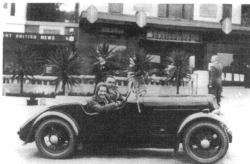
"Jack Bezzant navigates the actual two-seater special which has been discovered in Essex (BPC 796). Note the 30 louvres along the bonnet, no driver's door, the helmet cycle front wings with torpedo side lights, the position of the fold-flat windscreen supports, the twin wind cowls and the general shape of the elbow rests and tail."
