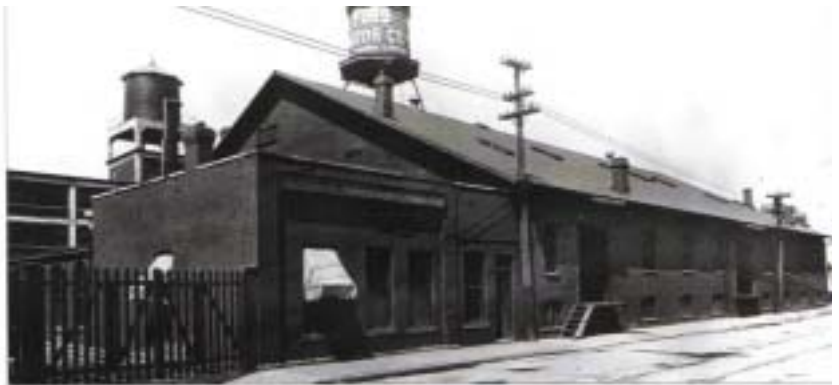
The Ford Motor Company of Canada Limited was born in this unassuming red brick building, formally known as the Walkerville Wagon Company, a builder of horse-drawn carriages.
