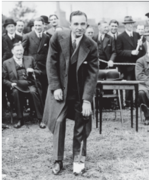
Edsel Ford cutting the first sod on the Essex marshes at Dagenham in 1929. Note the bent silver spade. It bent at Edsel's first attempt at digging!
