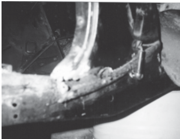
This shows the extent of the rot at the base of the off-side A post
