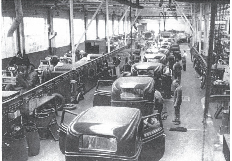
Having been carried down Kent Road five at a time on transporters from Briggs Bodies Ltd. to the main Ford plant at Dagenham, the Model 'Y' bodies were fed on to the High Line, where they were kitted out with trim, upholstery, wiring looms, instrumentation, etc. before being lowered onto chassis on the main production line.
