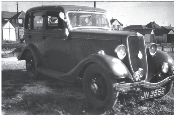
Christopher Hudson's uncle's Fordor Model 'Y', JN 3556, a late 1933 Southend-on-Sea registration. It was a long rad 1934 model and, being a Fordor, was the de luxe version, with (visible in the photograph) twin windscreen wipers, trafficators, rustless steel head lamp and sidelights and chromed windscreen surround. Note also the flat headlamp lens with the circular Magnaflex bars, which were introduced with the long rad in October 1933.
