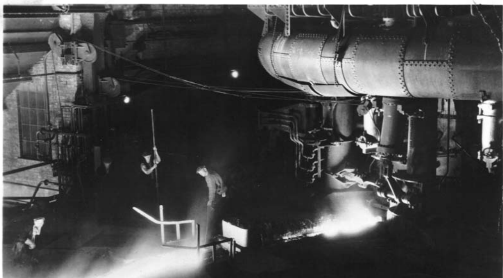
Hot work casting pig iron in the foundry.
