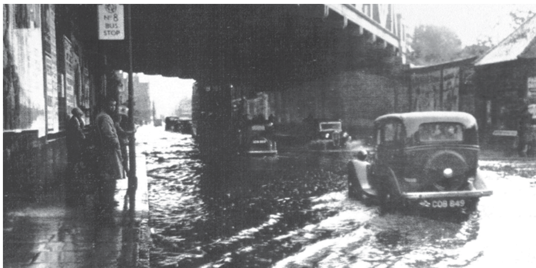
Dave Bond sent in this photograph of a 1936 Birmingham registered Tudor 'Popular', COB 849, chasing an Austin Ruby through the floods on Chepstow Road, Newport, then in Monmouthshire in South Wales in the early 1950s
