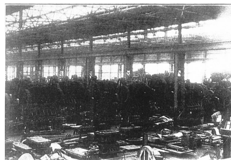
General view of the press shop
