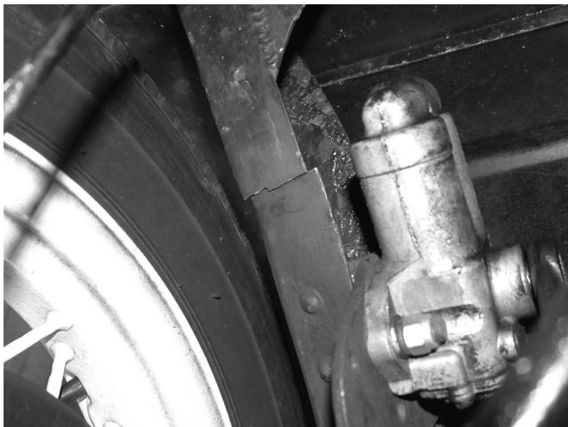
The oldest known Model "C" on the road has suffered a cracked chassis. John Keenan believes it is due to one of the many potholes following our hard winter.
