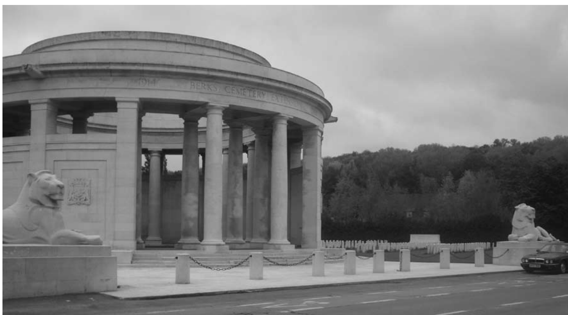
The Ploegsteert Memorial to the Missing sited on the Berkshire Cemetery Extension. The Last Post is sounded here every month. Note the size of the rotunda compared to the Jag parked by one of the lions.
