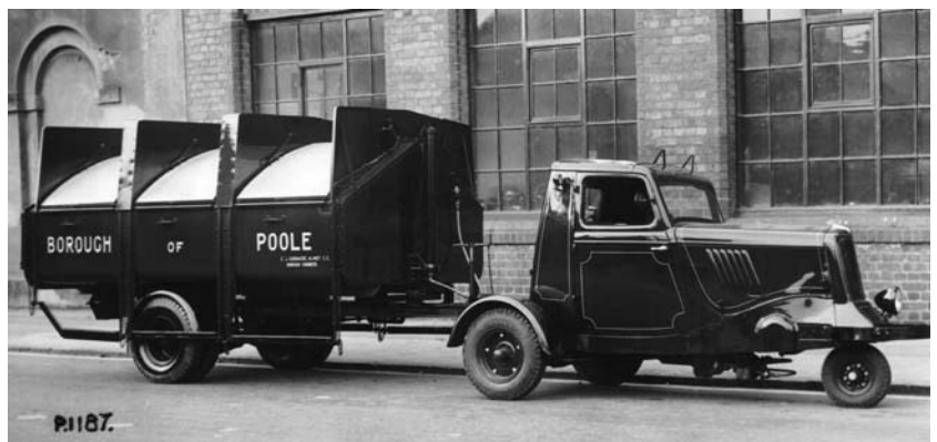
"A Borough of Poole refuse collection Tug with its automatic coupler to a bespoke trailer."
