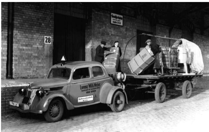
An Eifel Zugmaschine with its gear reduction ‘help-axle’ and reworked rear wings to accommodate the wider rear wheels’ track. Note that the car also has producer gas cylinders at the rear and wartime, shielded headlamps. The triangle above the windscreen indicates that the car is towing a trailer.
