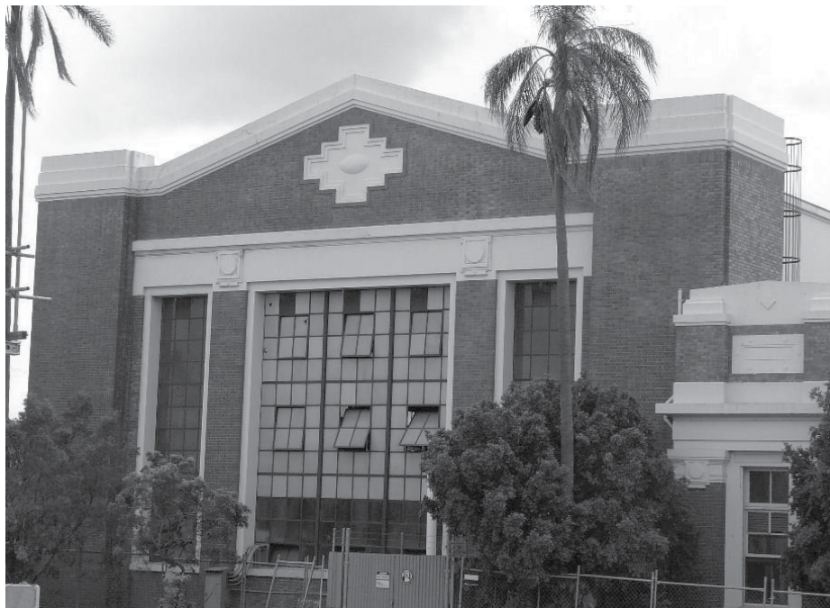
The typical Ford assembly plant art-deco exterior of the plant in Brisbane, Queensland. Photograph taken in 2008 whilst construction work was being undertaken by the then occupants, G. James Glass & Aluminium
