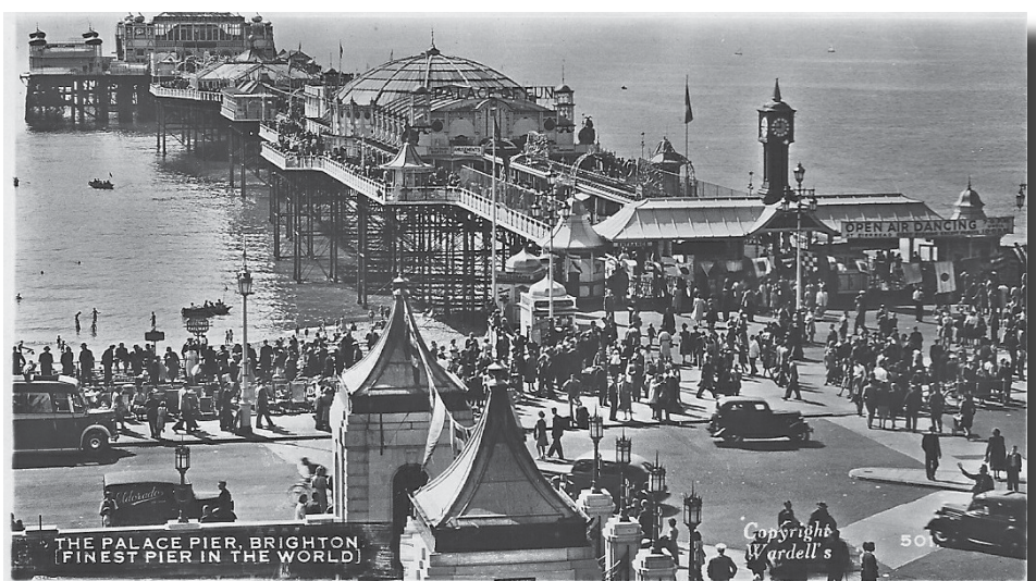
The stationary Tudor Model "Y" travelling west in front of the pier. The 'pedestrian on the crossing' by the Model "C" is a policeman directing the traffic.
