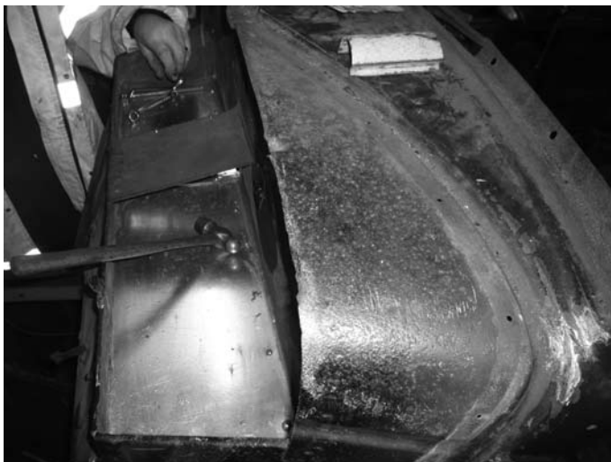
.... and here the tool and battery boxes
