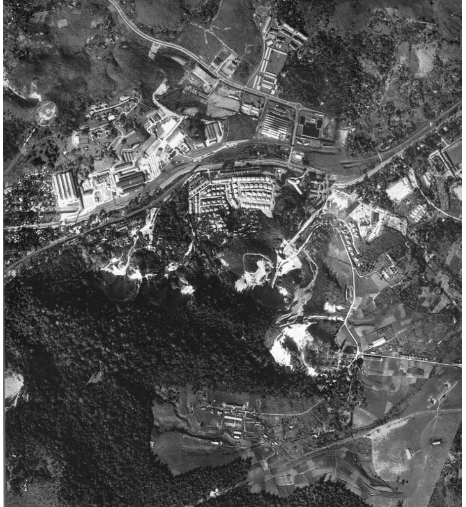
The aerial view of the Ford of Malaya plant on Bukit Timah Road in the 1950s. The assembly plant was in the four long sheds to the left of the photograph. Singapore city is to the left along the main road which, to the right, goes north to the Causeway and Johore Bahru, Malaya.
