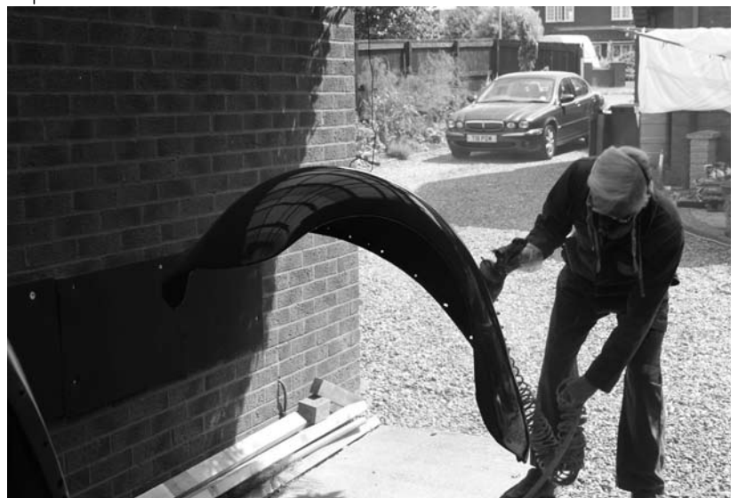
Spraying the top maroon coats. [I'm delighted to see that Bob has retained the maroon colour, which the tourer had when owned by the late Geoff Murrell – Ed.]
