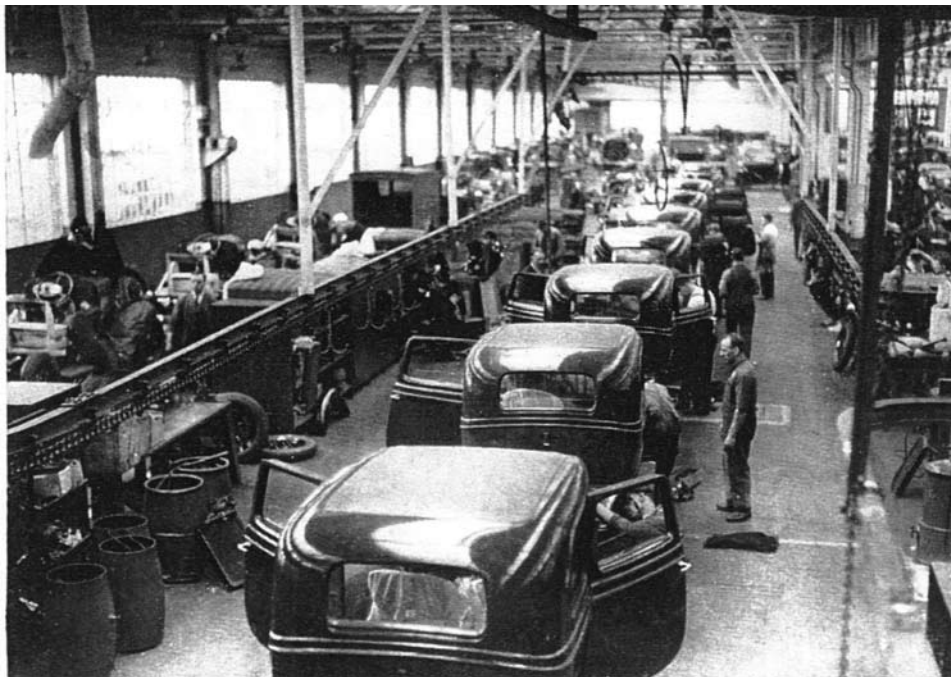
The 'High Line' which ran above the main production line. Here we see the Briggs body-shells being kitted out.
