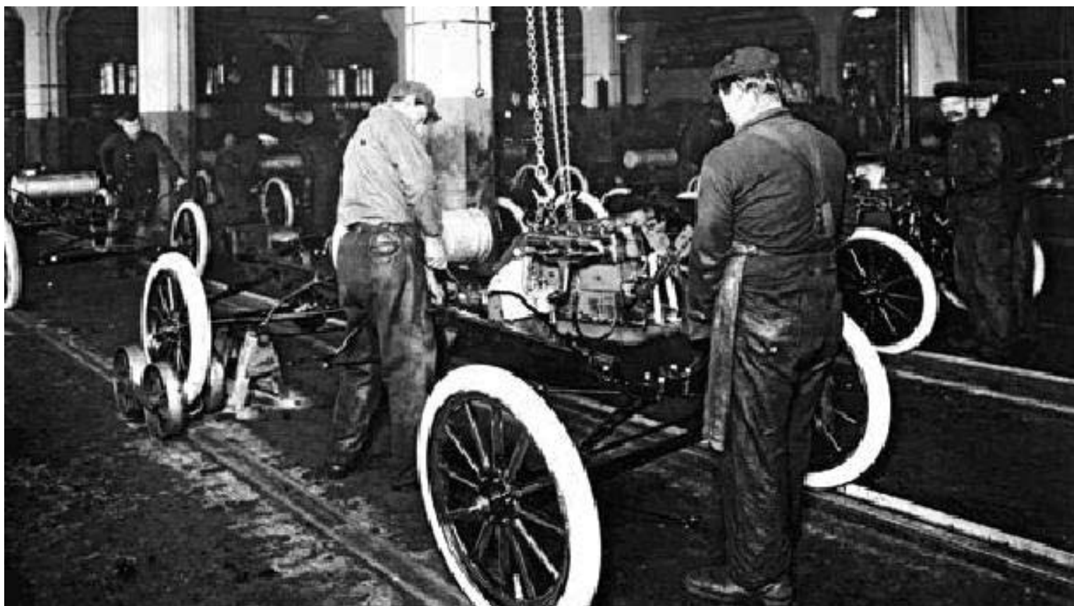
"The first moving assembly line at Highland Park, Detroit, using a rope to pull cradles carrying Model T chassis along a track."
