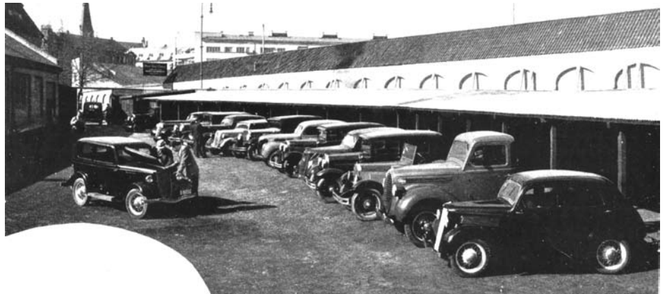
A Tudor Model "Y" (Ford Junior) appears to have been brought in by its owner and is having its engine looked at by a technician. A Model "C" Fordor (Ford Junior De Luxe) sits in the repair
