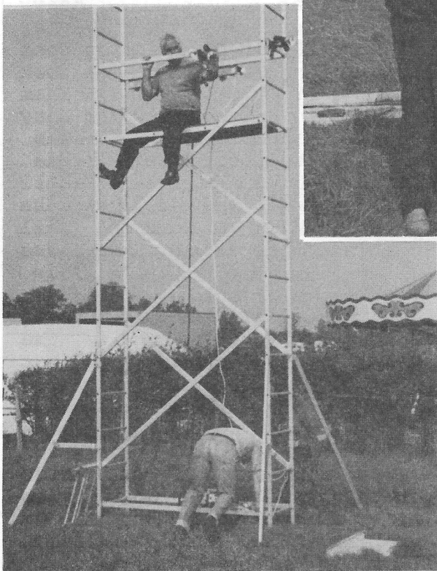
Graham and Peter on scaffolding.
